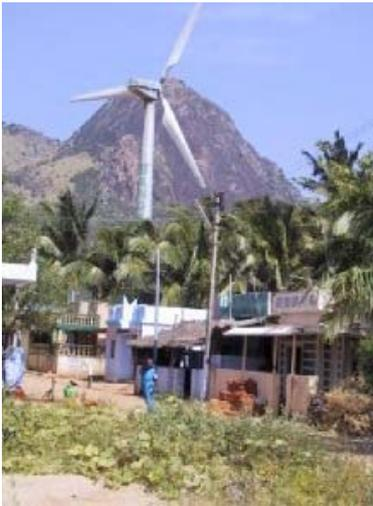
Visited the flat Muppanthal Valley on the tip of Southern India in Tamil Nadu State and travelled through many kilometres of wind turbines. These generators are small by modern standards but are currently being assessed to upgrade their capacity. There is a total wind generation of 1200MW in the valley alone.
