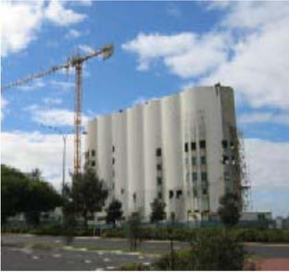
A development currently being undertaken in Bunbury is the conversion of the cement grain silos into housing units. This may be an option for silos in South Australia where they become redundant.
